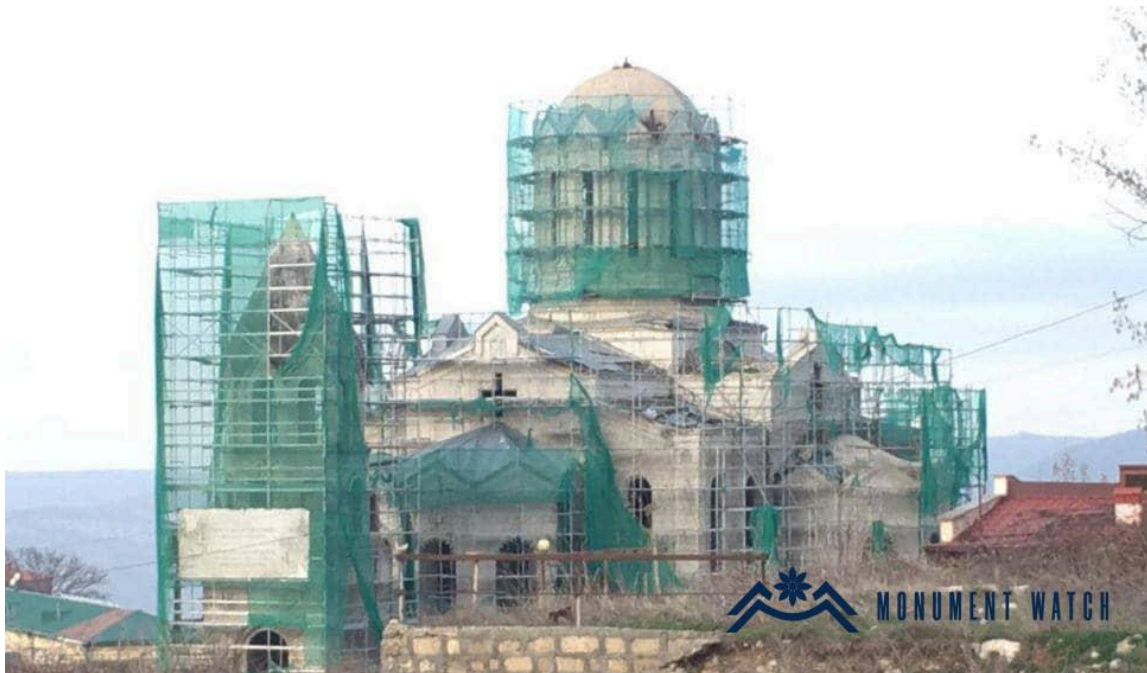
Figure 4 28 - The “restored” state of the Ghazanchetsots Church under Azerbaijani occupation
